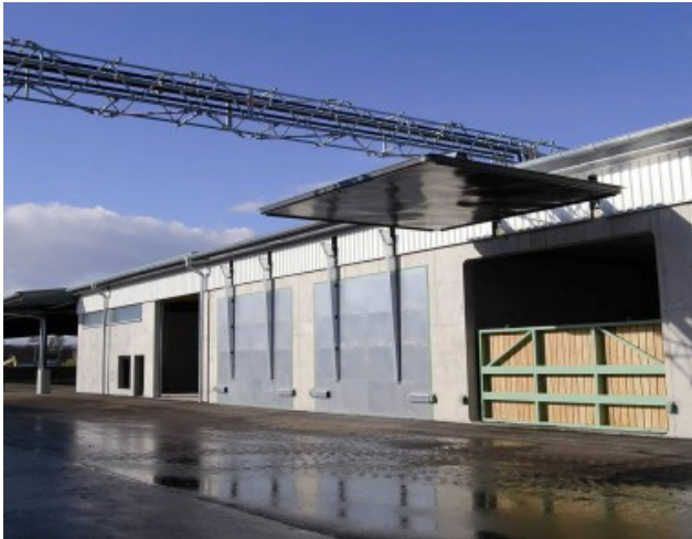
Figure 3. Air tight bay doors of BEKON reactors in open and closed positions (from www.bekon.eu ).
